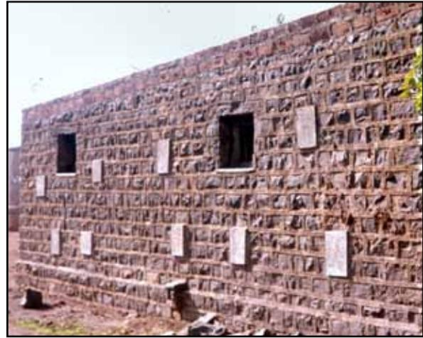
Figure 4.20: Examples of completed through-stone retrofit projects in Maharashtra, India (photos: S. Brzev)
