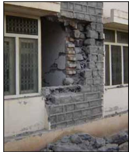
**Figure 2.38** Vertical cracking at a wall intersection in the 2005 Kashmir, Pakistan, earthquake due to absence of connection between the intersecting walls, a stone masonry and a brick-masonry wall (source: Bothara and Hiçyılmaz 2008)
