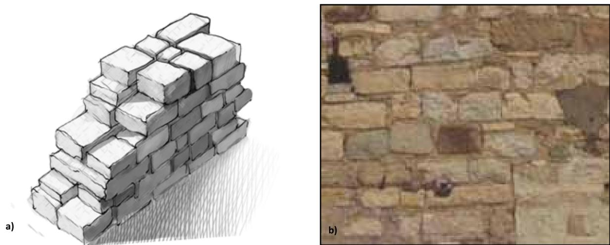
**Figure 1.31** Dressed stone masonry: a) an isometric view of a typical wall, and b) an exterior of a wall in Umbria, Italy (source: Maffei et al. 2006)
