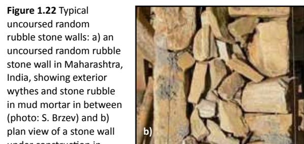
**Figure 1.22** Typical uncoursed random rubble stone walls: a) an uncoursed random rubble stone wall in Maharashtra, India, showing exterior wythes and stone rubble in mud mortar in between (photo: S. Brzev) and b) plan view of a stone wall under construction in Nepal (note stone rubble between the wall wythes) (photo: Smart Shelter Foundation)
