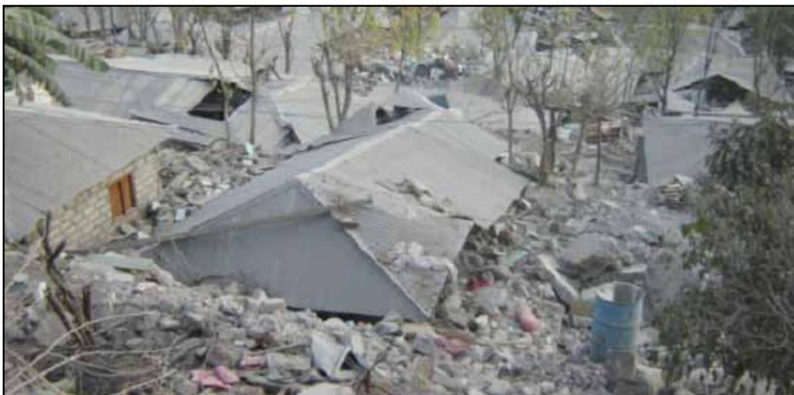
**Figure 2.17** Collapse of stone masonry buildings with hipped roofs in the 2005 Kashmir, Pakistan, earthquake (source: Bothara and Hiçyılmaz 2008)
