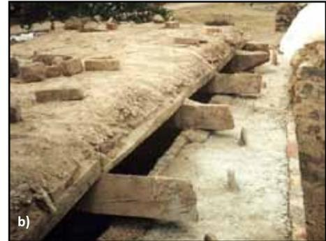
**Figure 4.6** An example of a field application of an RC band in an existing stone masonry building in Maharashtra, India: a) RC band installation completed (note brick edging at the band level and a newly constructed portion of the wall above the band), and b) RC band at the roof level underneath the timber beams (note that the roof is supported by an interior timber frame) (photos: S. Brzev)
