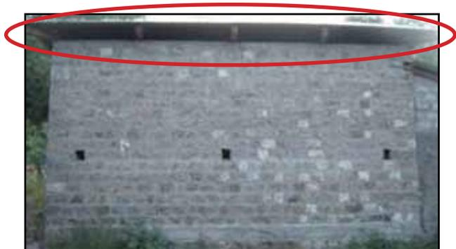
**Figure 2.10** A stone masonry building in Muzaffarabad was undamaged in the 2005 Kashmir, Pakistan, earthquake; this was attributed to the presence of an RC band at the eaves level (photo: J. Bothara)
