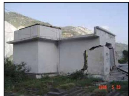
**Figure 2.39** Soil spreading in the 2005 Kashmir, Pakistan, earthquake - note wide cracks in the walls (source: Bothara and Hiçyılmaz 2008)
